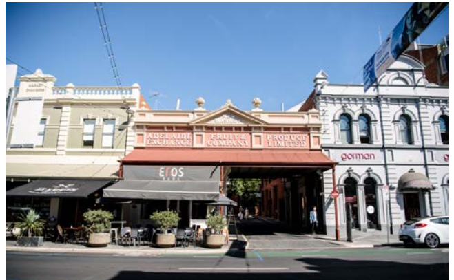
Heritage shop frontages
