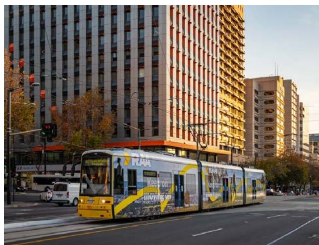
North Terrace Tram
