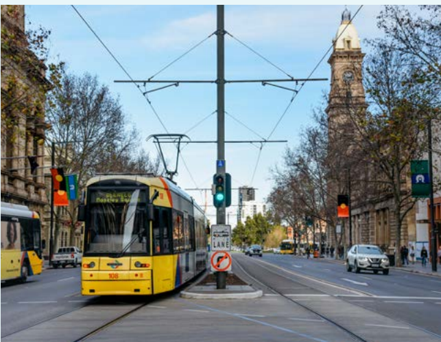
King William Street tram connection
